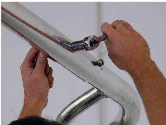
Once all the holes are drilled and all the fasteners are inserted (M10 x 75mm - Button Head Socket Bolt) the nylon lock nuts can be installed and all of the fasteners and nuts can be firmly tightened.
