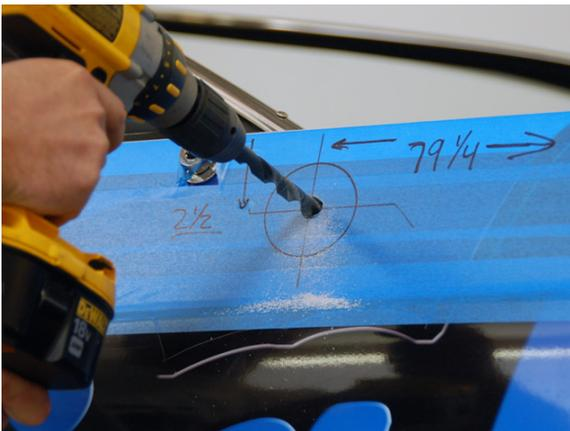
If necessary, you should move the wires out of the way while you drill. We recommend drilling a small pilot hole which will keep the 17/32" drill bit from walking (moving). A small rat tail file can be used to ease the edge and keep the gel coat from chipping. Be careful of wires!
